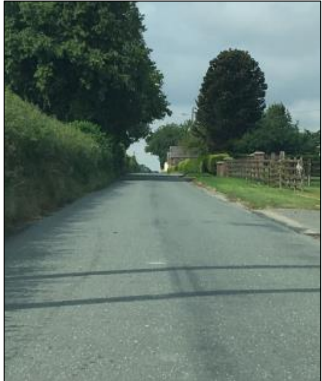
Image 28-9: L-2226 (west of the skew bridge).
