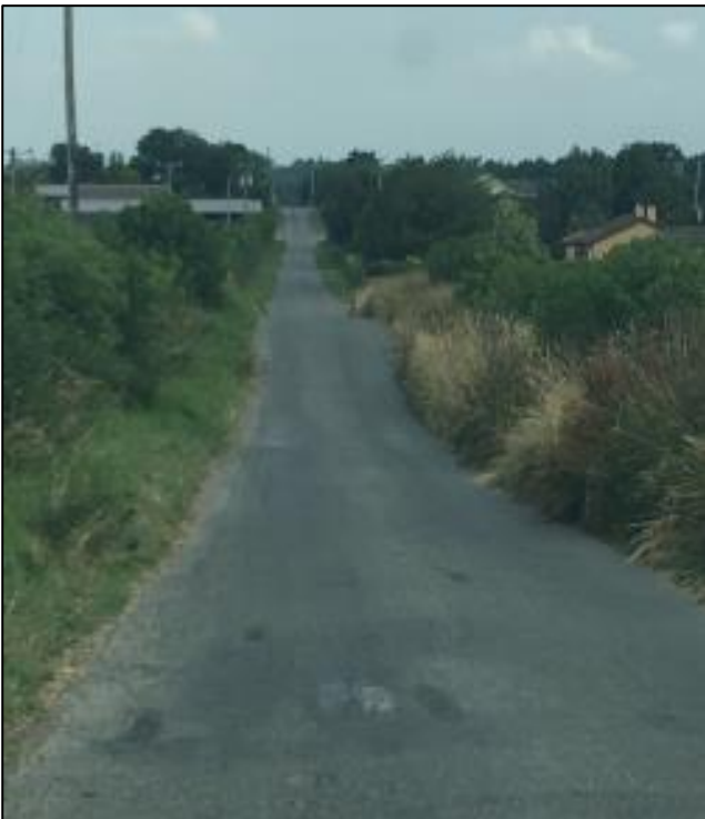
Image 28-14: Undulating Vertical Alignment.
